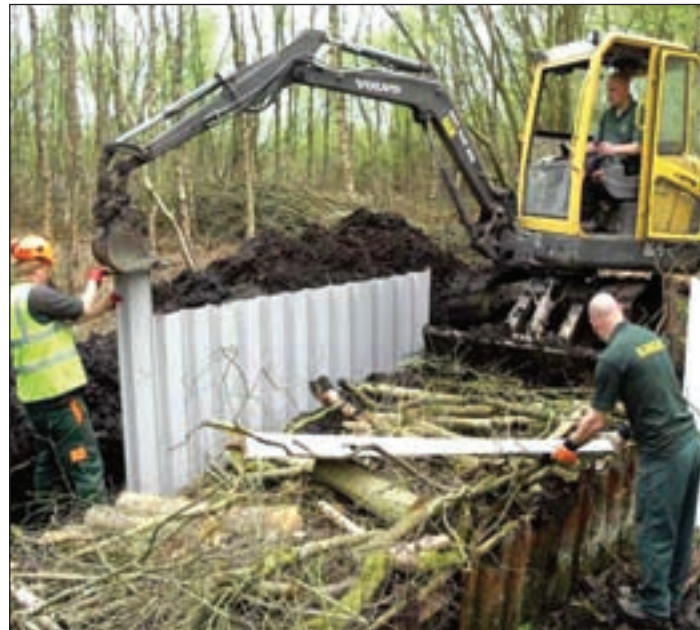
Construction work: Plastic piling is keyed into the bank.
