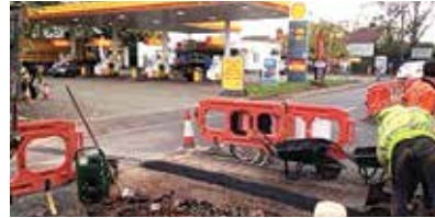
The scene in Higher Lane as the work was carried out.
